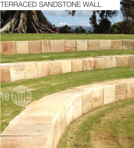
TERRACED SANDSTONE WALL
